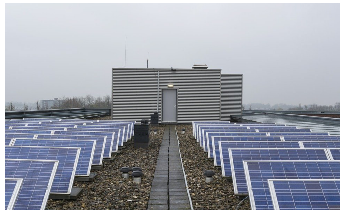
Figure 1. Battery energy storage system linked to solar array. Source: Pixabay
