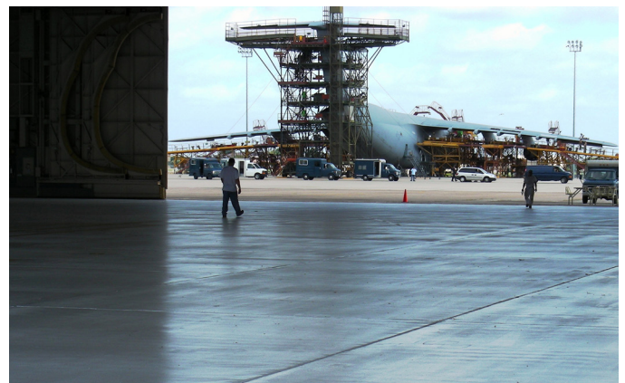
Figure 2. U.S. military hangar with highly reflective paint to aid aircraft inspection. Source: 433 AW
